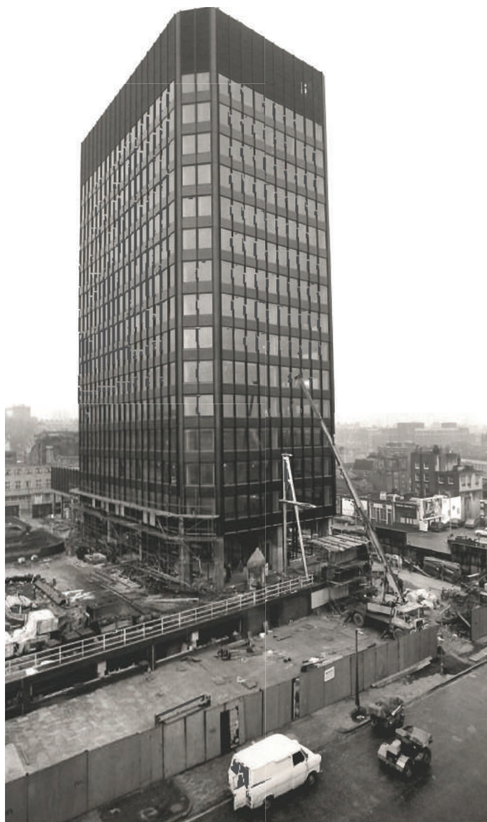
Phase 1 of Kings Cross House, before construction of the second tower 6
