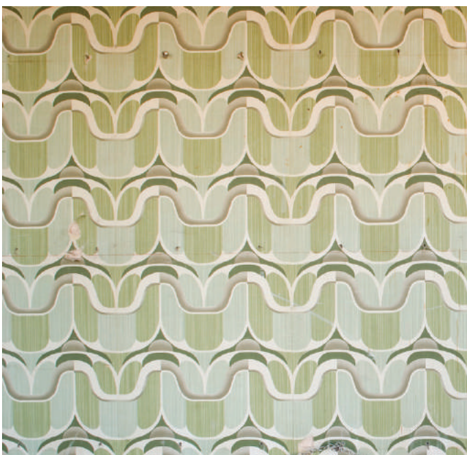
Top floor canteen wallpaper - possible survivor of the original fit-out 8
