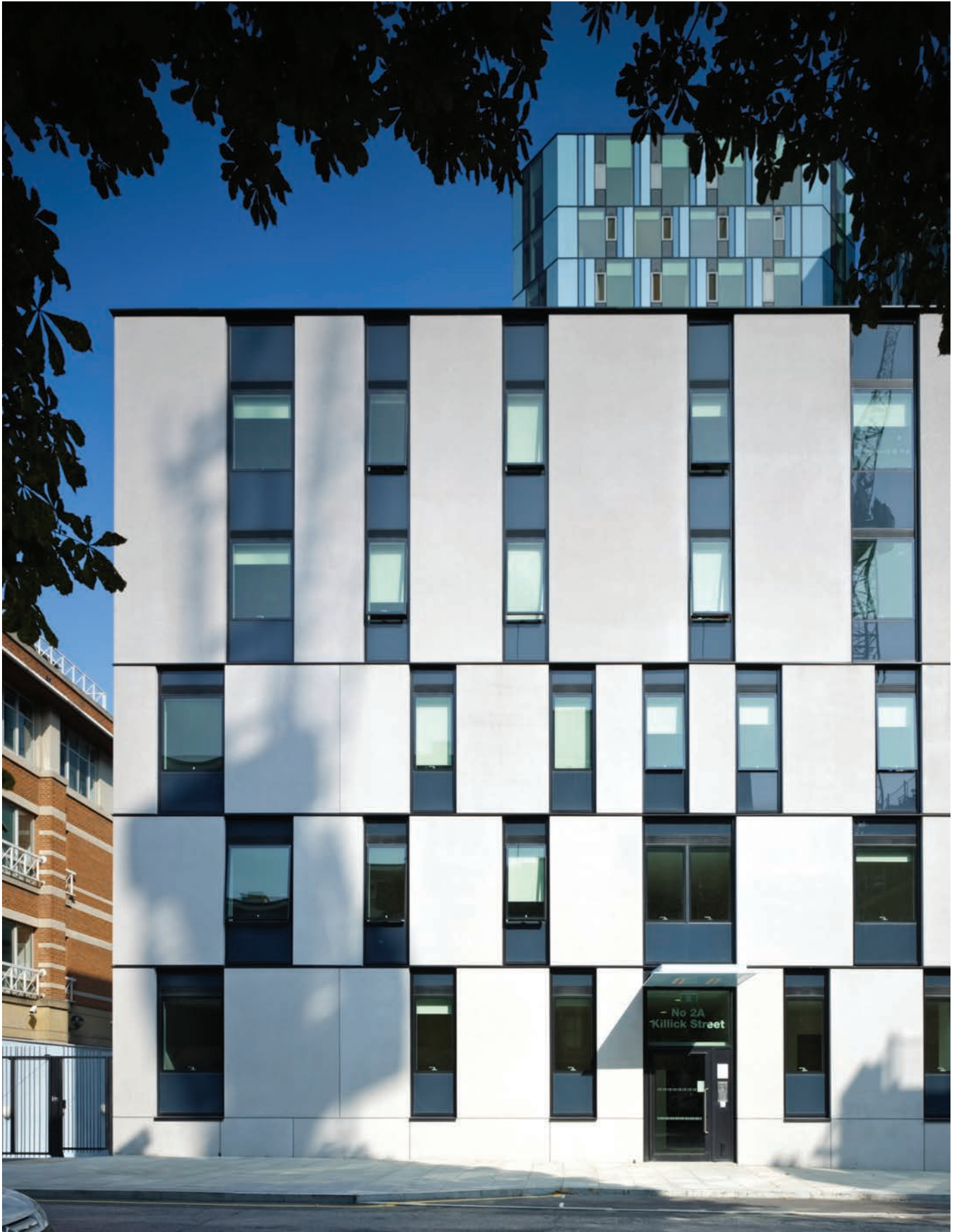
Detail of tower concrete cladding, linking the passing street to the building
