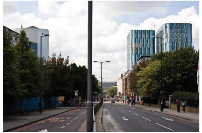
Newly clad towers nearing completion
